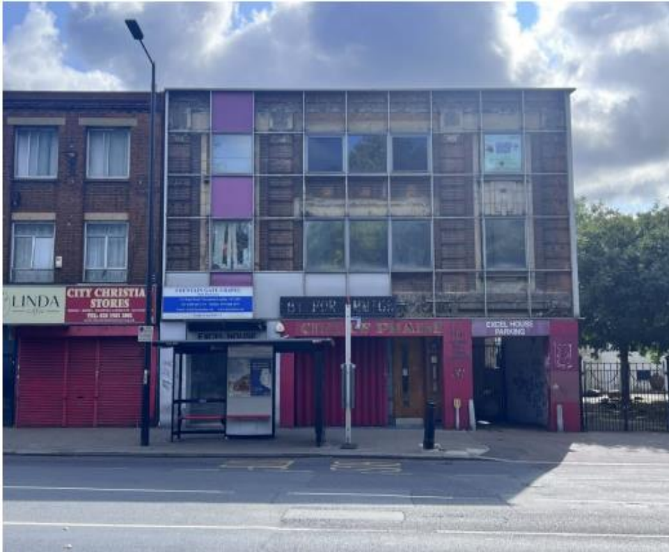
Extant front elevation with most cladding removed.
